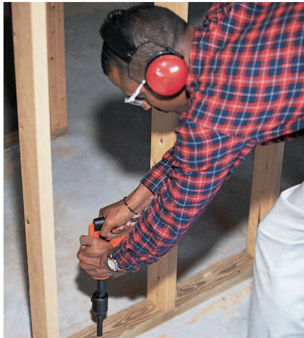
Figure 3-8 Powder-Actuated Tools Proper Protection Powder-actuated tools are powerful. Hearing and eye protection are essential when using them. Never use this tool unless you have been trained in its use.
