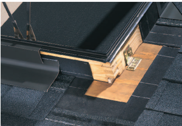
Figure 20-20 Curb-Type Skylight Properly Flashed Some skylights rest on a wood curb. The curb may be supplied by the skylight manufacturer, as shown here, or it may be constructed on site from 2×6 lumber.
