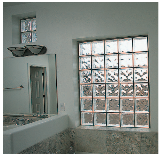
Figure 20-6 Glass Block Strong and Private Glass blocks can be used to admit light where ventilation is not required.
