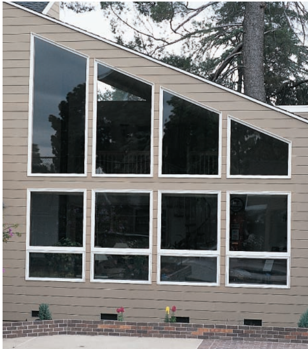
Figure 20-4 Fixed and Awning Windows Two Types of Windows The top row consists of stationary windows. The bottom row consists of stationary windows above smaller awning windows.
