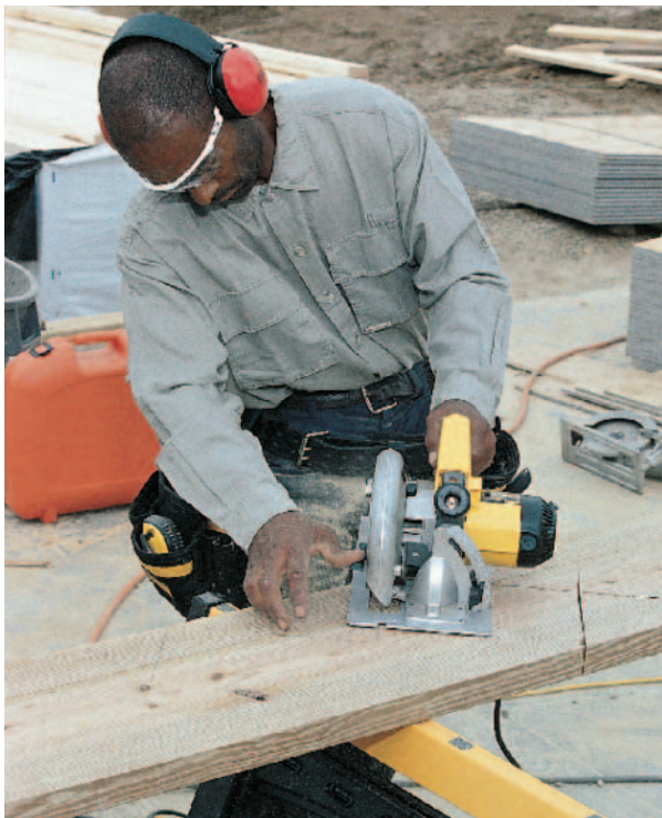
Figure 25-18 Cutting the Stringer Two Saws With the stringer resting on sawhorses, use a circular saw to cut just along the layout lines. A. To avoid overcutting, use a handsaw or jigsaw to finish the cut. B. Why should overcutting be avoided?
