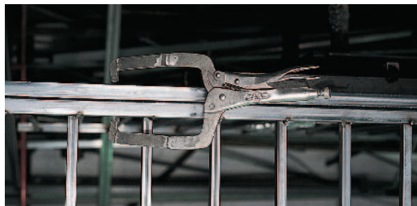
Figure 29-13 Locking C-Clamps Prevent Jacking These clamps temporarily hold members together.
