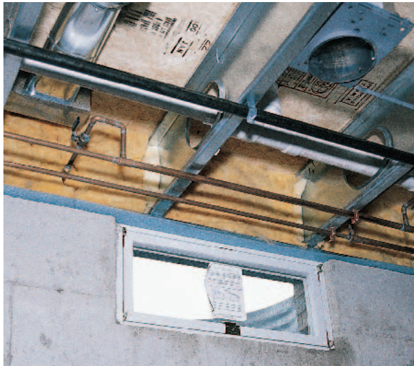
Figure 29-23 Basement Foundation Steel Joist A basement foundation with steel floor joists in place.
