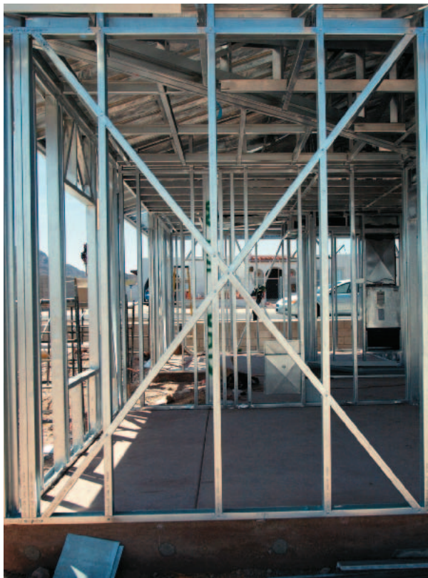
Figure 29-45 Bracing Diagonal Support X-bracing using steel straps.
