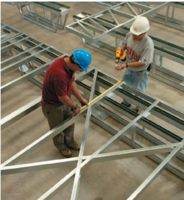
Figure 29-2 Panelization Table Pre-Built Panels can be built to exact specifications and tolerances.
