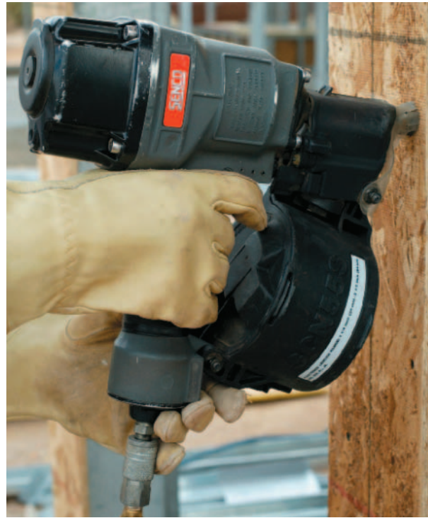
Figure 29-7 Nailer Attaching Sheathing A nailer used to attach sheathing to steel studs.
