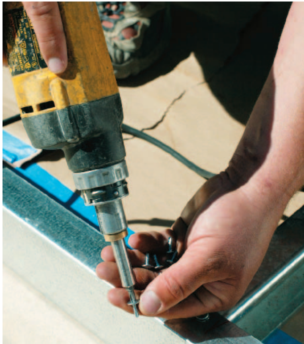
Figure 29-3 Feathering Screws Attaching Screws Feathering screws with a power screw gun.
