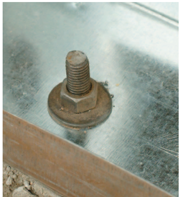
Figure 29-29 Anchor Bolt Anchored Embedded anchor bolt.
