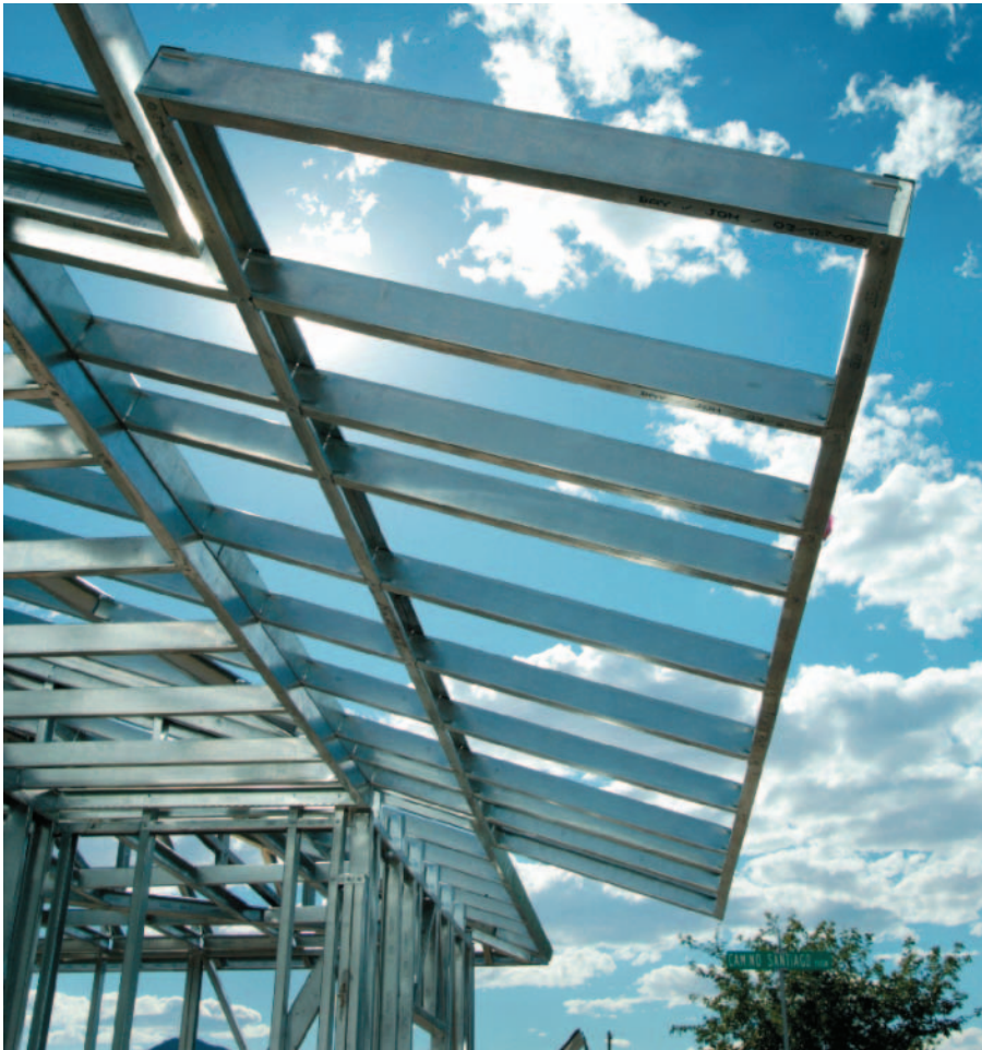
Figure 29-55 Lookouts Extra Support Lookouts can be used to form a rake.
