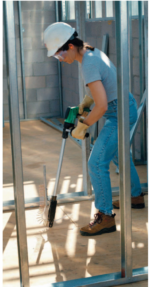
Figure 29-5 Drill Attachment Remain Standing This drill attachment drives collated screws. It allows the worker to stand while drilling. After this worker positions the tool, she will straighten it to a perpendicular position. Screws should always be driven perpendicular to the floor sheathing.
