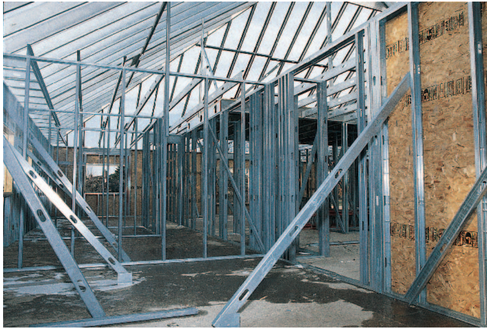
Figure 29-35 Braced Walls Proper Support Temporary wall bracing.
