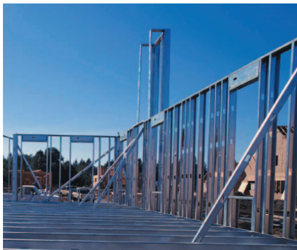
Figure 29-40 Panelized Walls Pre-Assembled Sections These panelized wall sections were built on a flat surface.
