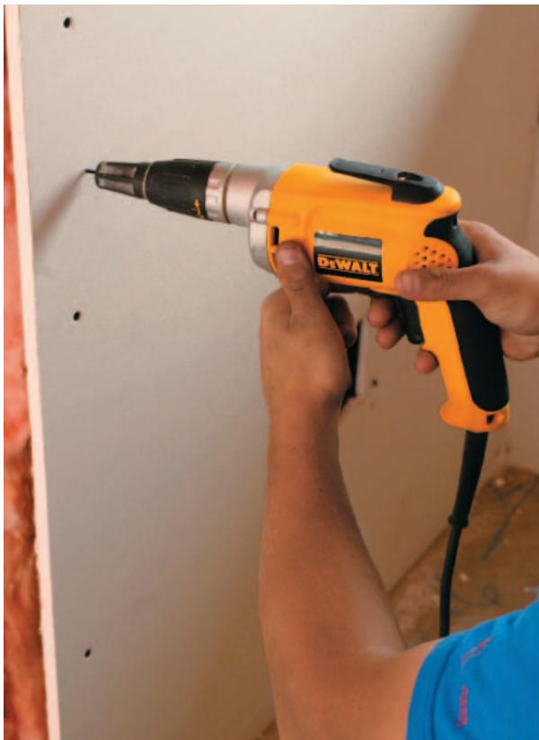
Figure 29-6 Drywall Screw Gun Protecting Sheathing A drywall screw gun has a depth-sensitive nosepiece.
