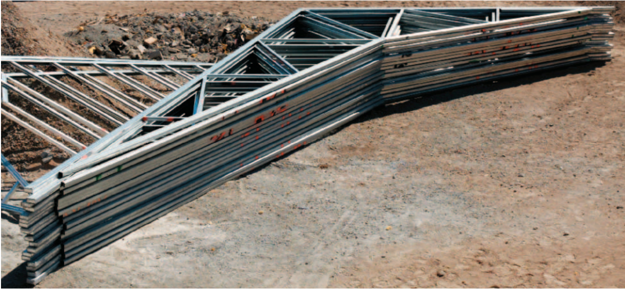
Figure 29-49 Roof Trusses No Gussets Roof trusses are built in many styles and shapes.
