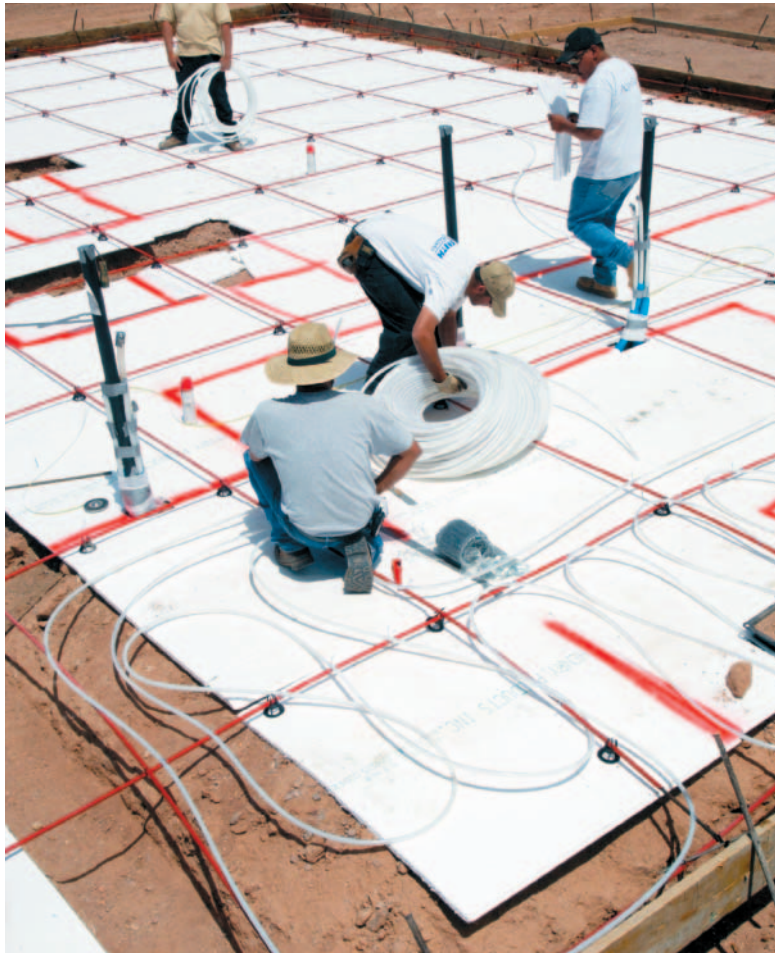
Figure 30-21 Preparing for Radiant Heat
