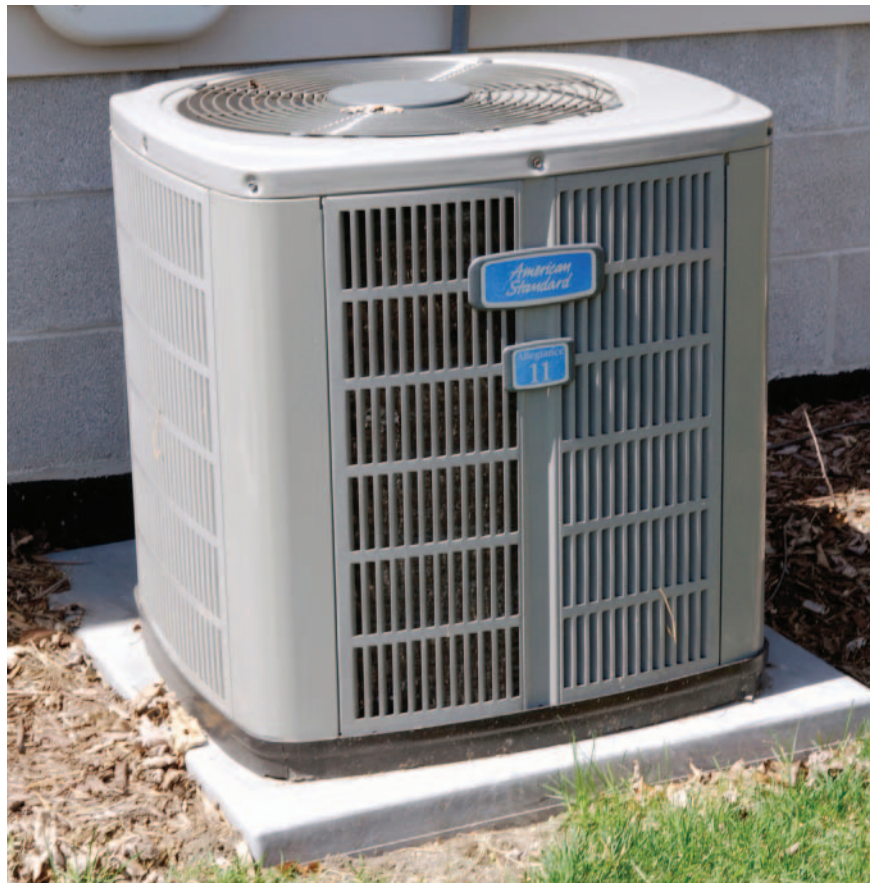
Figure 30-19 Heat Pump
