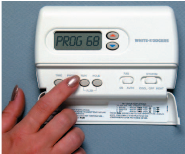
Figure 30-16 Electronic Thermostat Programmable Electronic thermostats can be set to change temperatures on an hourly or daily basis. They are sometimes called set-back thermostats .
