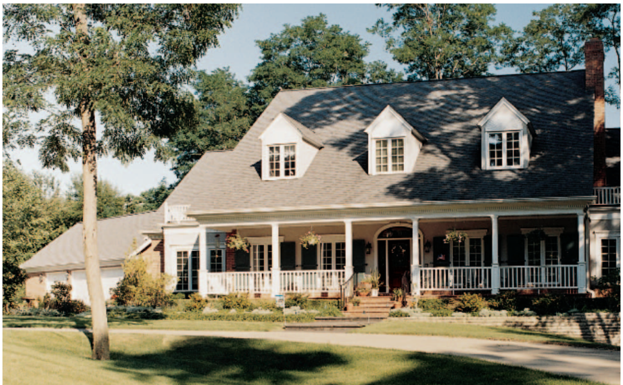
Figure 35-15 Full-Length Entry Porch
