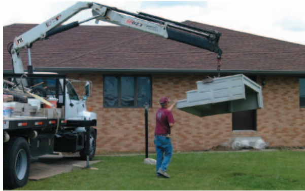
Figure 35-17 Precast Steps Ready to Use Precast step units are hollow to reduce weight. However, they are still heavy enough to require placement by crane.
